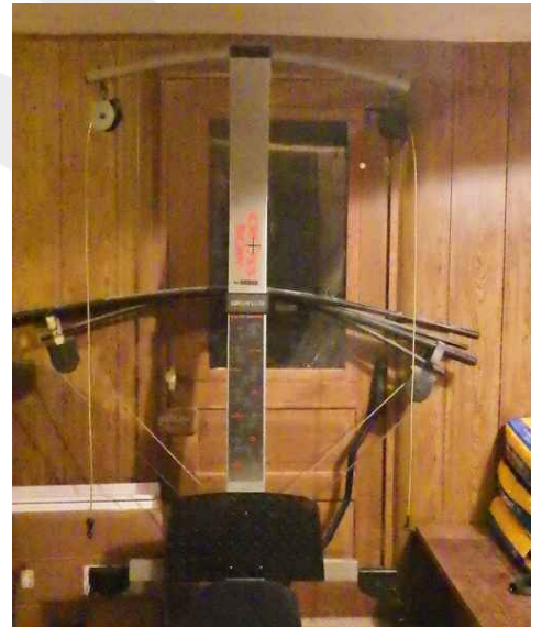
Exercise machine blocking emergency egress door in basement
