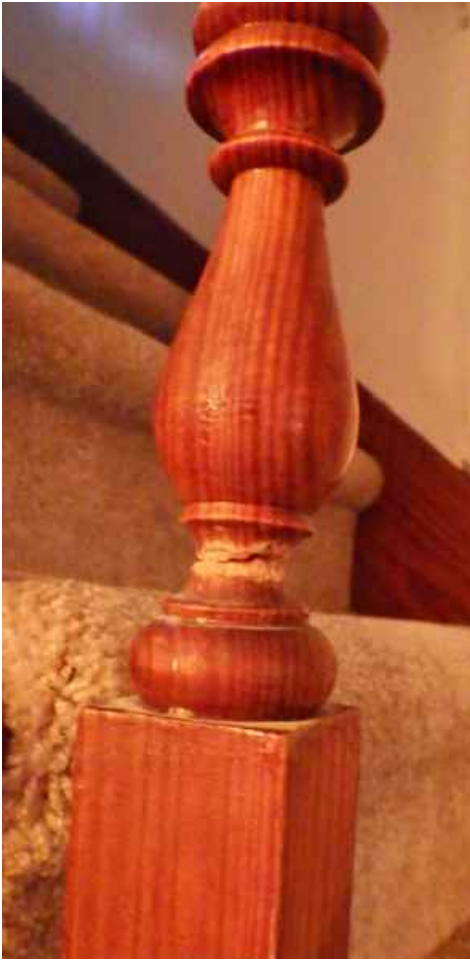
Damaged spindle.
