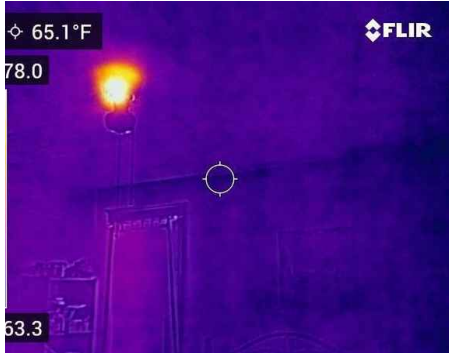
Exterior window and fan generating heat.
