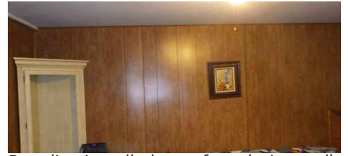
Paneling installed over foundation wall.
