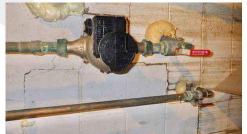
Cracking in brick foundation at mortar joints, shows past evidence of water intrusion. Does not seem to be recent.
